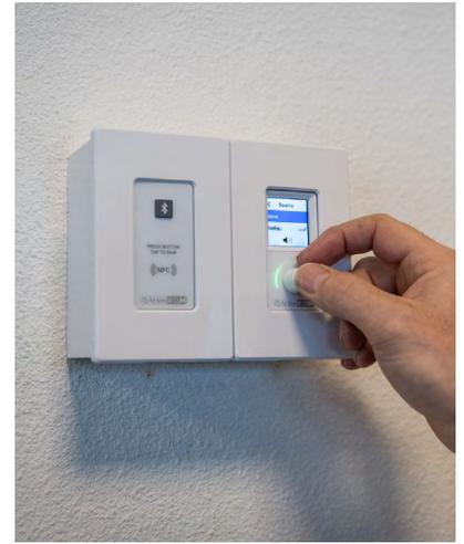
**MULTIPLE C-ZSV ZONE SOURCE AND VOLUME WALL CONTROLLERS WERE INSTALLED IN THE SPACE, WITH VITAL LIMITATIONS IN PLACE TO DEFINE THE FEATURES EMPLOYEES COULD USE AND WHICH NEEDED TO BE LEFT TO THE PROFESSIONALS.**
